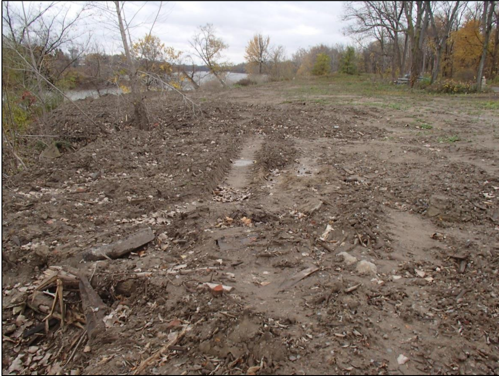
Photo 9: View from the southwest edge of pit toward fresh grading, facing southwest.
