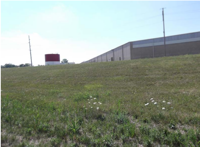
Photo 17 – Looking southeast toward Campbell's Plant from southern portion of project area.
